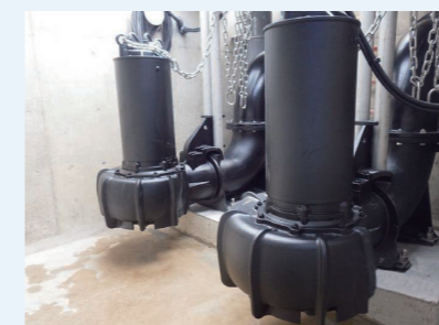
Large-scale submersible pumps for road drainage systems (pump bore of 400 mm x 22 kW in power)
