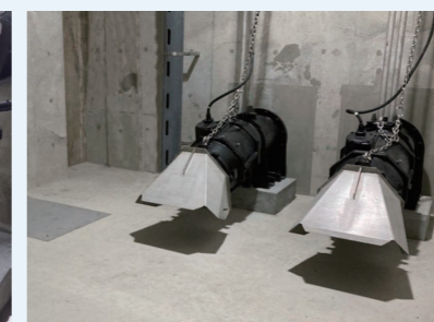
Large-scale horizontal-shaft submersible pump for rainwater storage facilities (pump bore of 500 mm x 11 kW in power)
