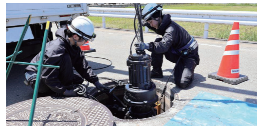
■ Maintenance being conducted by ShinMaywa Aqua Technology Service, Ltd.
