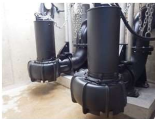
Large-scale submersible pumps for road drainage systems (pump diameter of 400 mm x 22 kW in power)
