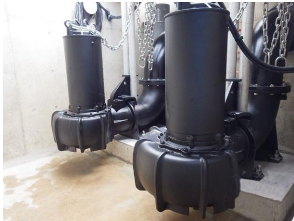
Large-scale submersible pumps for road drainage systems (pump diameter of 400 mm x 22 kW in power)
