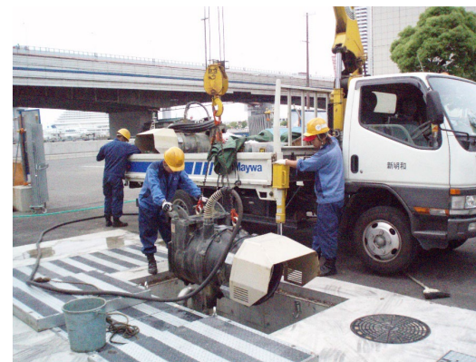
K City Rainwater drainage pumps (horizontal axial-flow)
