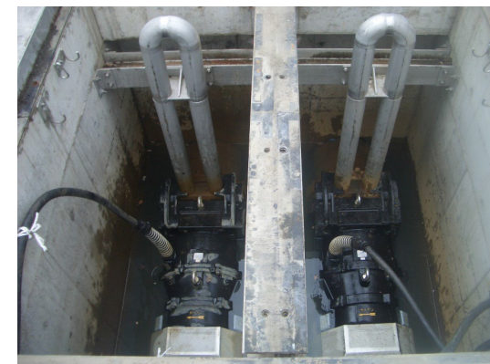
K City Rainwater drainage pumps (horizontal axial-flow)
