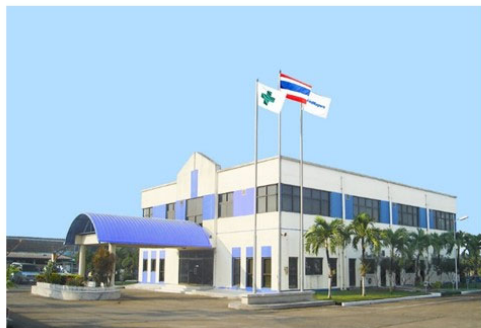
Production base in Thailand (Thai ShinMaywa Co., Ltd.)
