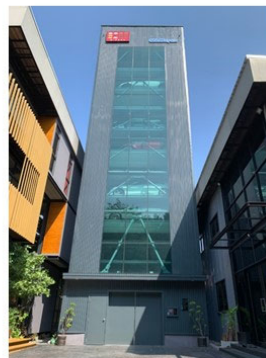
Showroom-specification parking facility completed on the premises of G-PARK "G-PARK & ShinMaywa Tower"
