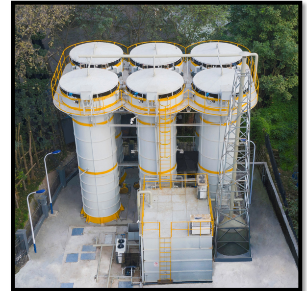
Promoting waste water treatment business at a newly established local subsidiary in China (Photo shows equipment delivered to Chongqing city)
