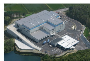
Refuse Transfer Station System
