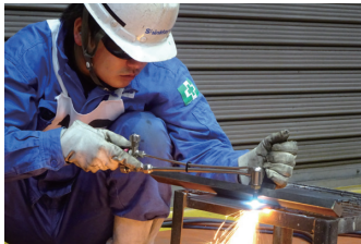
Competition at Hiroshima Plant (structural steelwork)
