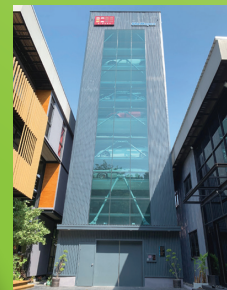
Mechanical car parking system showroom (Bangkok, Thailand)
