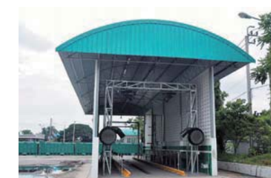
Car Washing Building with Automatic Washing System
