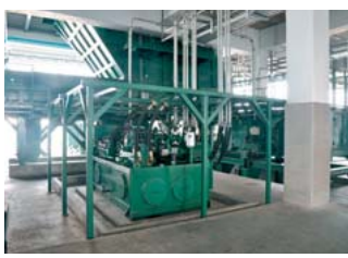
Hydraulic Power Unit
