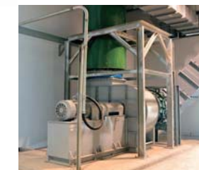
Odor & Dust Control System (Fan)
