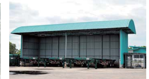
Container Washing Building with Manual High Pressure Washing
