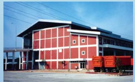
Jakarta Refuse Transfer Station (Indonesia)
