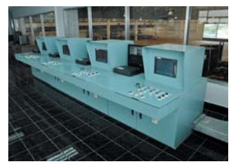
Central Control Room
