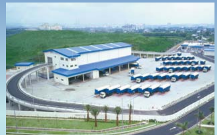
Kuala Lumpur Refuse Transfer Station (Malaysia)
