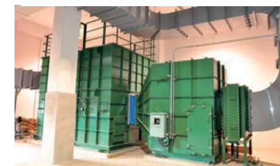
Odor & Dust Control System (Filter & Absorber)
