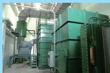
Odor & Dust Control System
