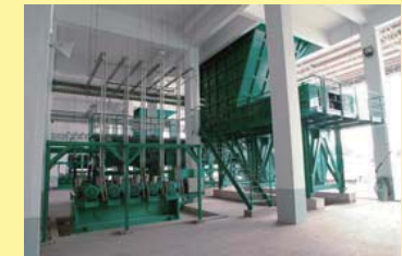
Hydraulic Power Unit
