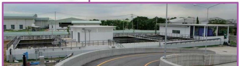
Water Treatment Building
