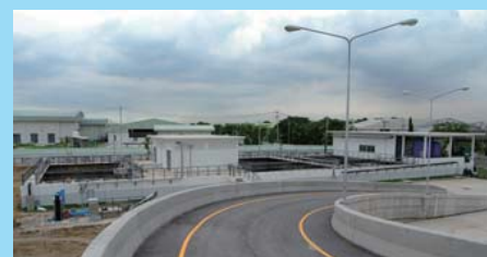
Water Treatment Building
