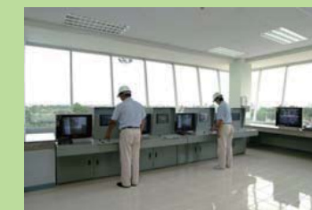
Central Control Room
