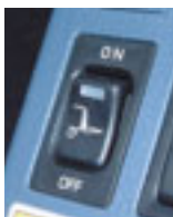
Main switch inside the cabin
