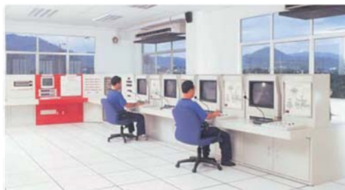
● Central Control Room
