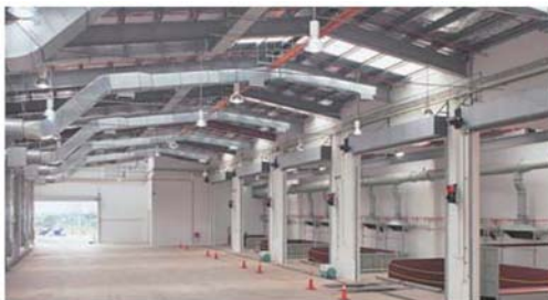
● Unloading Area (2nd Floor)
