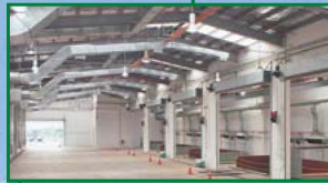
● Unloading Area (2nd Floor)
