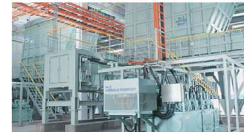
● Compactor System (Ground Floor)
