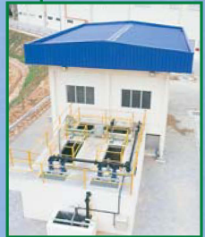
● Leachate Treatment Plant
