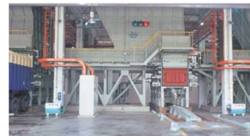
● Compactor System (Ground Floor)
