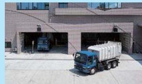
Shinjuku Refuse Transfer Station, Tokyo
