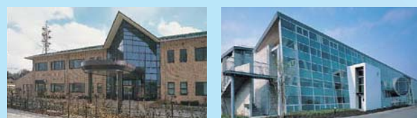
Western Tottori Public Administration Recycling Plaza
